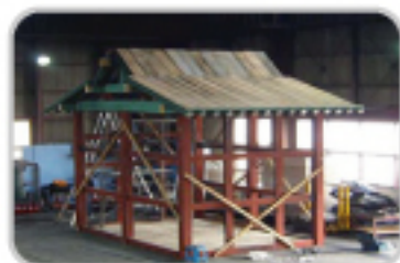
Mock-up for Fire Test
