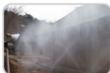
Installation Case of Shell type Water Curtain Nozzle
